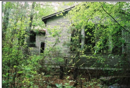
Page 225: Sims School: left-hand side of north front elevation with industrial room's bank of windows.
