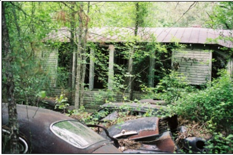
Page 223: Sims School: bank of window openings for west classroom at south rear elevation.
