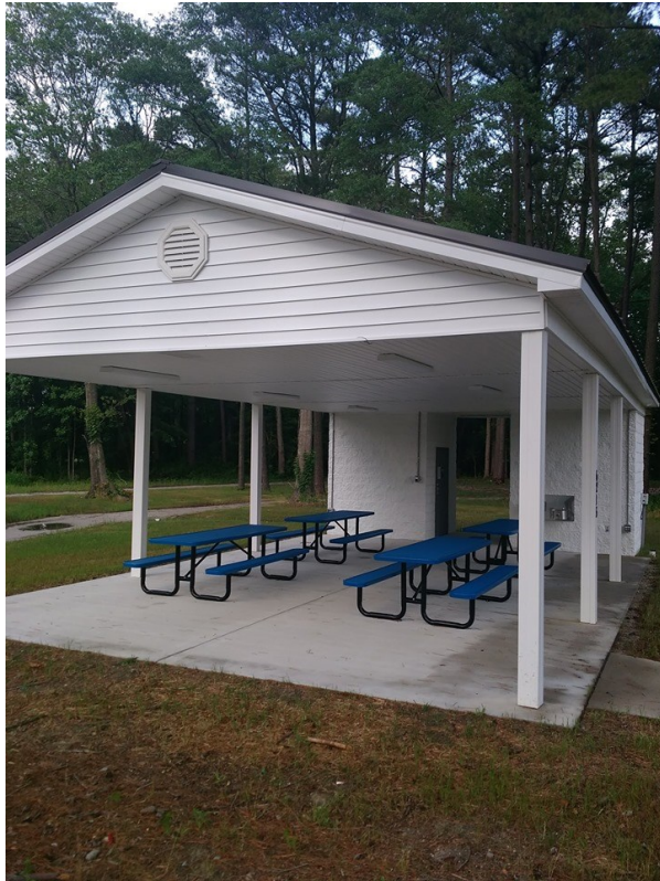
New Shelter at Sims Community Park
